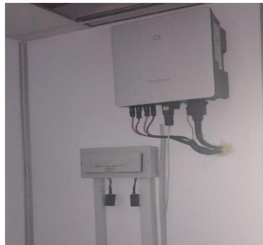
**Figure 3. Solar PV inverter**
